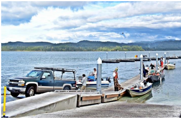
New Double Ramp Boat Launch
